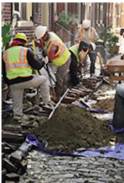
Work on American Street
